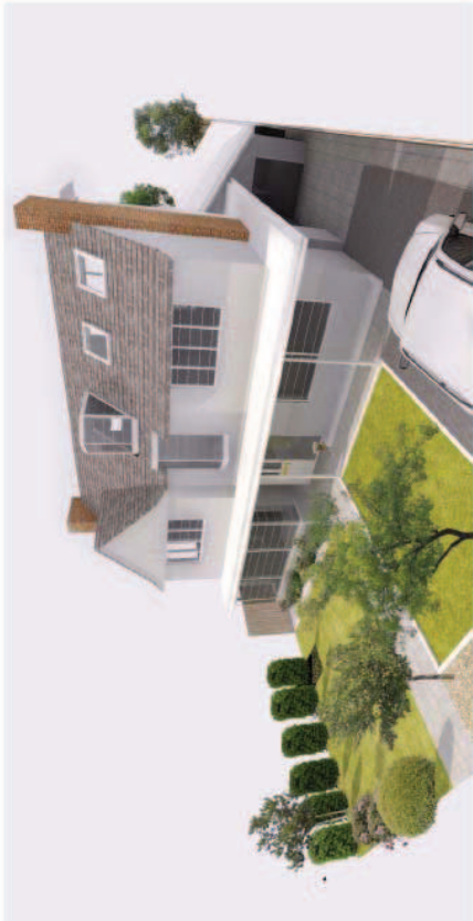
Above: Canopy on south facade provides shading from high sun at peak times of the day.
